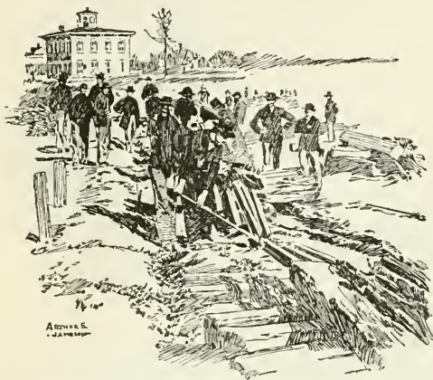
DESTROYING A RAILROAD AT ATLANTA, GA.
